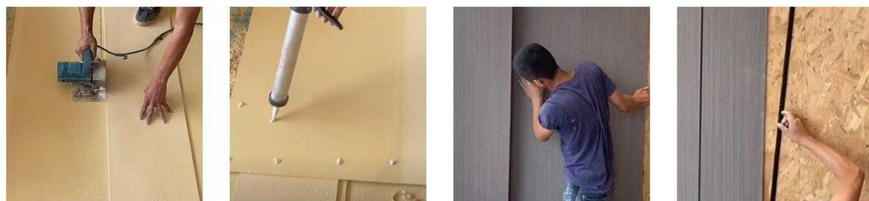
Step 1: Cut the WPC foam board to size. Step 2: Apply no-nail free glue to the back. Step 3: Install on the wall. Step 4: Insert the dovetail strips.
