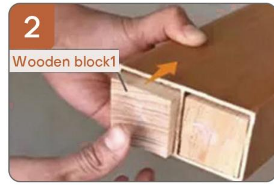
2.Insert the wooden block 1 which is 5cm in both ends of WPC timber tube.
