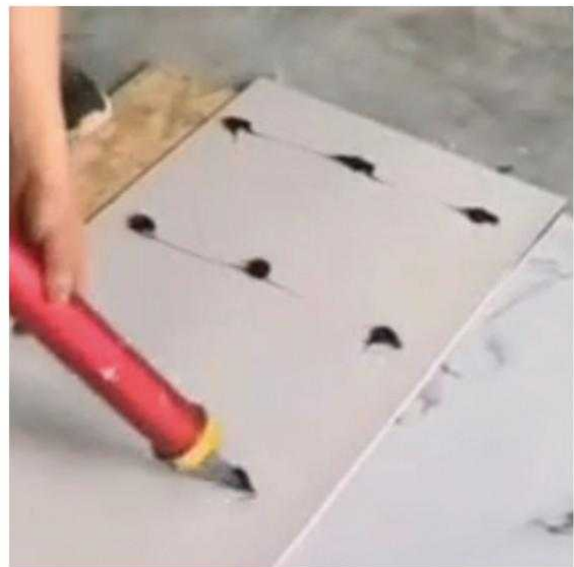
◦ Step 3 Apply nail free glue to the back.
