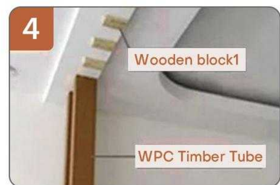
4.Fix wooden block 2 on position of the ceiling floor by glue, and then put the WPC square tube on the position of wooden block 2, then finish.
